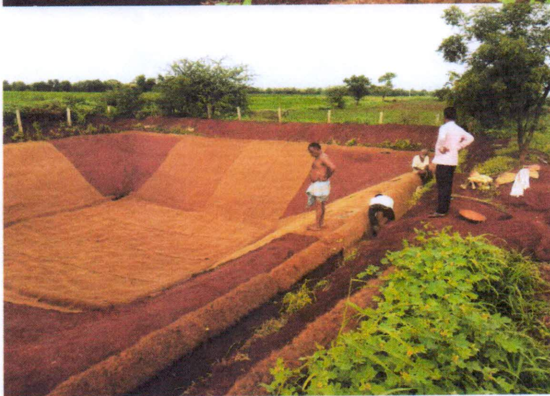
Picture 2. Farm pond is under construction using coir geo-textiles
